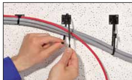
Q Ties can be used for temporary and final cable assembly.
