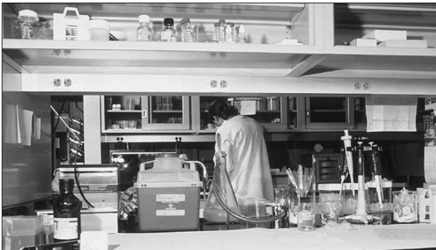
Standard devices installed in aluminum raceway mounted under reagent shelf in medical center lab.
