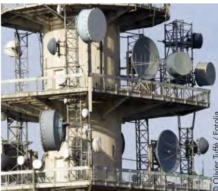
Telecom - Data infrastructure
