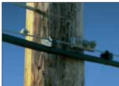
PANDUIT® cable ties and spacers are used to separate the support strand from the cable or to separate two cables in aerial lashing applications.
