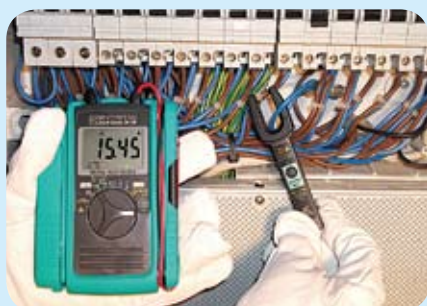
Measuring current in a Switchboard
