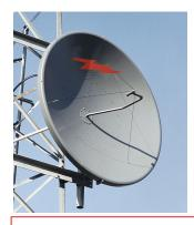
2.4 m | 8 ft Standard Parabolic Unshielded Antenna, single-polarized, 10.200–10.700 GHz, CPR90G, gray antenna, molded gray radome with flash, standard pack—one-piece reflector
