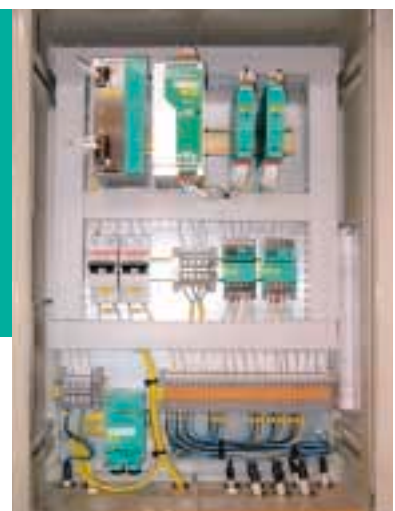
Switch cabinet with AS-Interface
