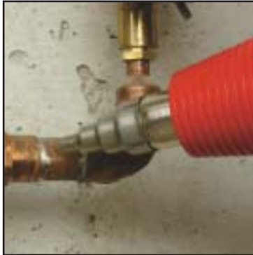
Solder Copper Pipe
