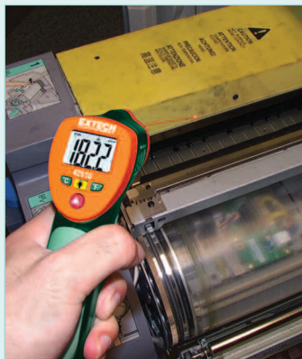
Electrical Troubleshooting for hot spot detection
