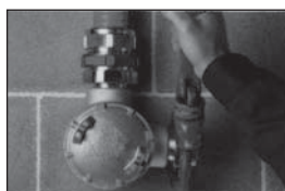
5. Install hub on enclosure
