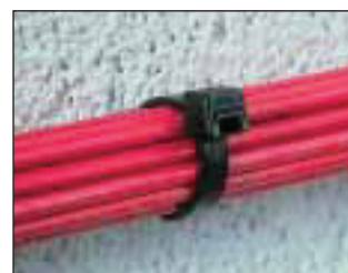
4. Install wires or cable.
