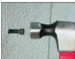
2. Hammer mount into hole.
