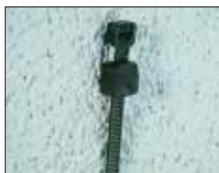
3. Place cable tie through mount.
