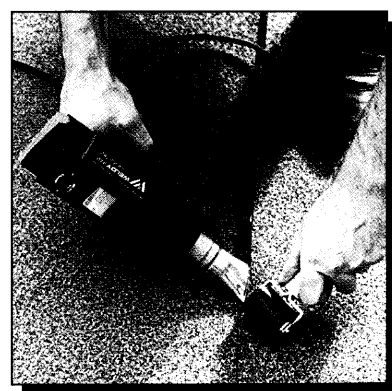
Welding bitumen and roofing felt
