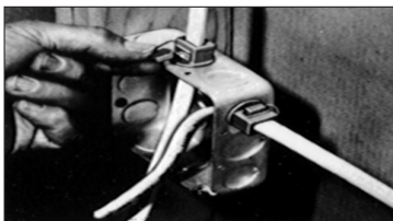
Snap captive locking wedge into connector's cavity.
