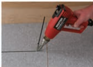
Welding Flooring Material
