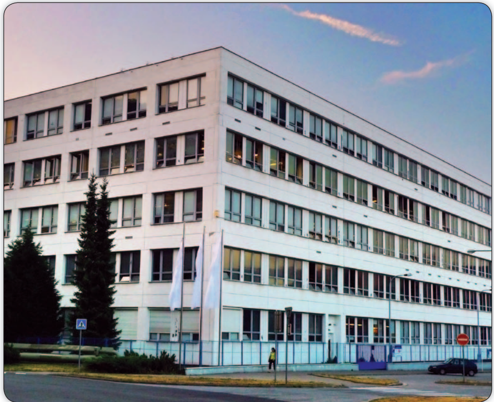
TE Manufacturing Facility in Trutnov, Czech Republic
