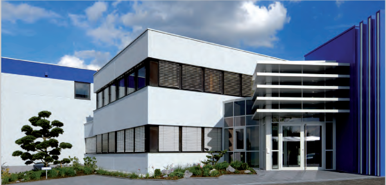
foyer of the company
