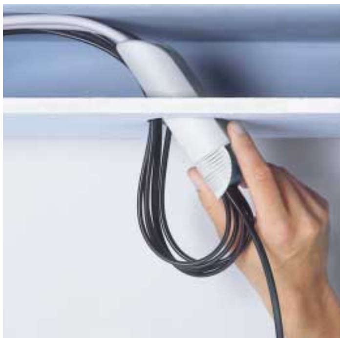
The wired-up 150 W Mouse is inserted, primary side first, in the ceiling opening.
