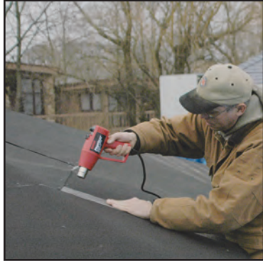
Weld Roofing Membrane
