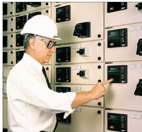
One MM2 is typically mounted in each starter of a motor control center.
