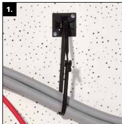
1. Insert tail and pull back towards the head.
