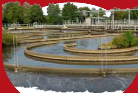
Waste Water Treatment
