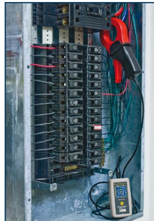
L101 recording branch circuit current.
