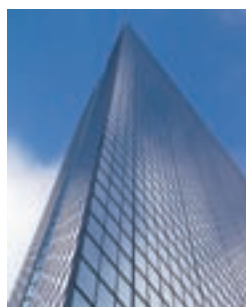
HVAC / Building management
