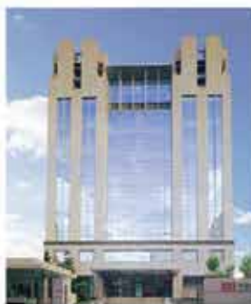
MEAN WELL GUANGZHOU TIANHE R&D CENTER
