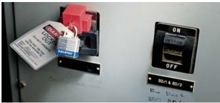
Oversized Breaker Lockout Device
