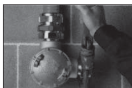
5. Install hub on enclosure
