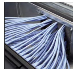
Firestop block adds protection to network wiring
