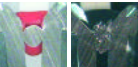
Photo 2 – Conductor insulation is pierced, first contact is made with the current bar.
