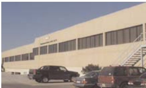
BCLM production facility
