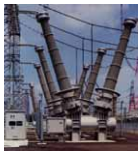
GAS switch gear (GCB/GIS)
