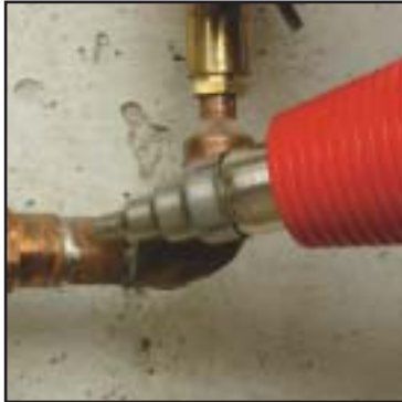
Solder Copper Pipe
