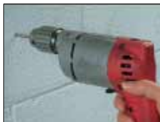
1. Drill hole using correct size bit.
