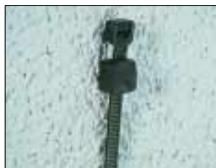
3. Place cable tie through mount.
