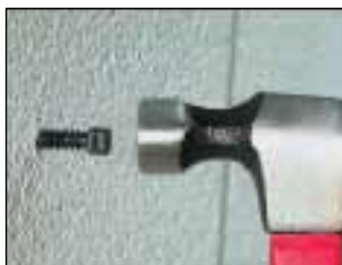
2. Hammer mount into hole.
