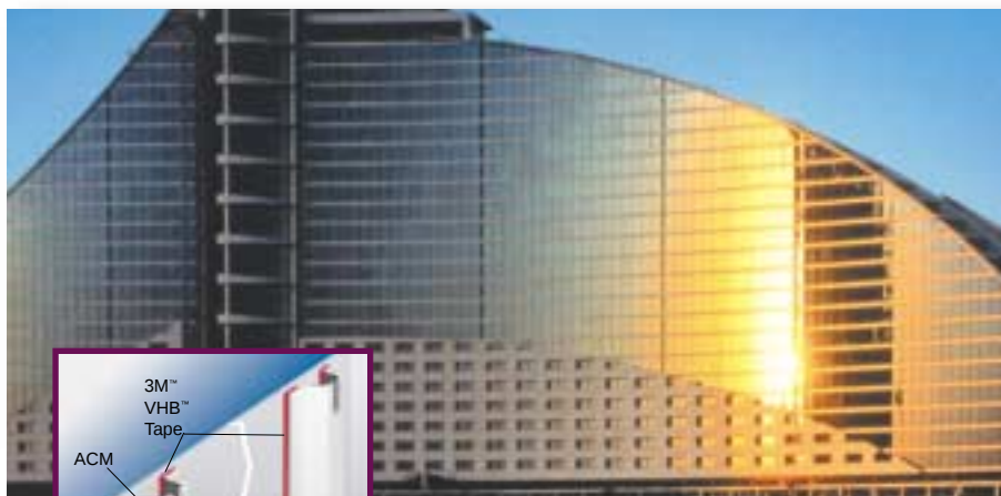
Jumeirah Beach Hotel, Dubai, UAE Curtain wall design: Schmidlin AG, 1998 Aluminum panels bonded to steel stiffeners.
