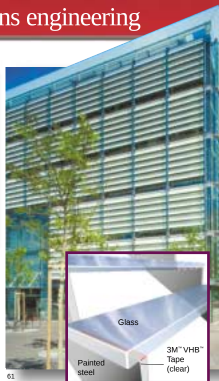
Glass steps bonded to varnished steel frame, Tamedia Building, Zurich, Switzerland
