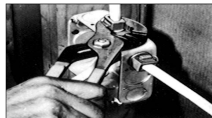
Press locking wedge into cavity which locks onto cable.
