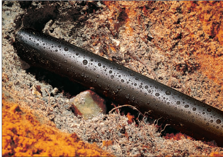
TREDUX HA47 - application below ground.
