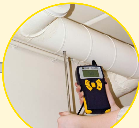
Ventilation duct inspection
