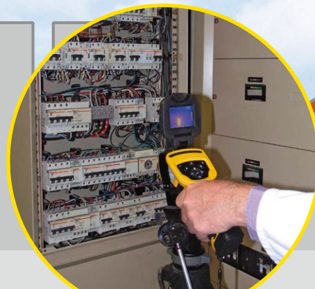
Inspection of electrical cabinets
