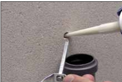
Fast-Bond - Bonding a pipe clamp anchor into aerated concrete
