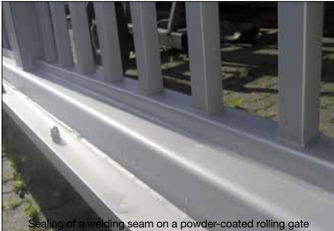
Sealing of a welding seam on a powder-coated rolling gate
