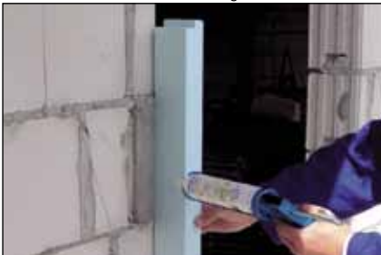
Fast-Bond - Bonding of hard foam panels on aerated concrete
