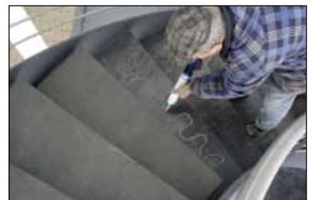
Flex 310 M Classic - Steel spiral staircase step (step plate of granite)
