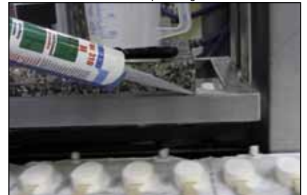
Flex 310 M Classic - Sealing on a filling plant in an ice-cream factory
