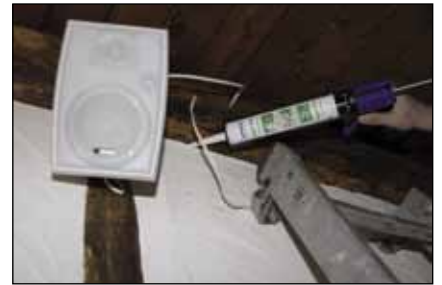
Flex 310 M Super-Tack - Fixing of lines
