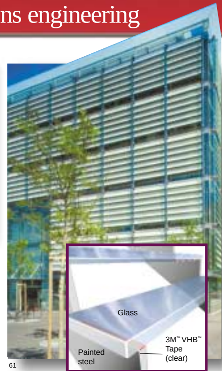
Glass steps bonded to varnished steel frame, Tamedia Building, Zurich, Switzerland
