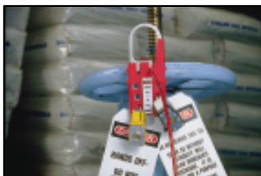
Gate Valve Lockout Device
