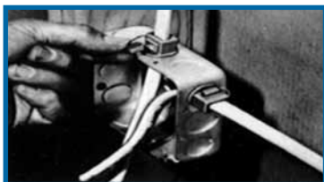
Snap captive locking wedge into connector's cavity.
