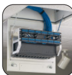
Zone Cable Boxes
