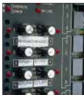
Label switches, relays and other devices
