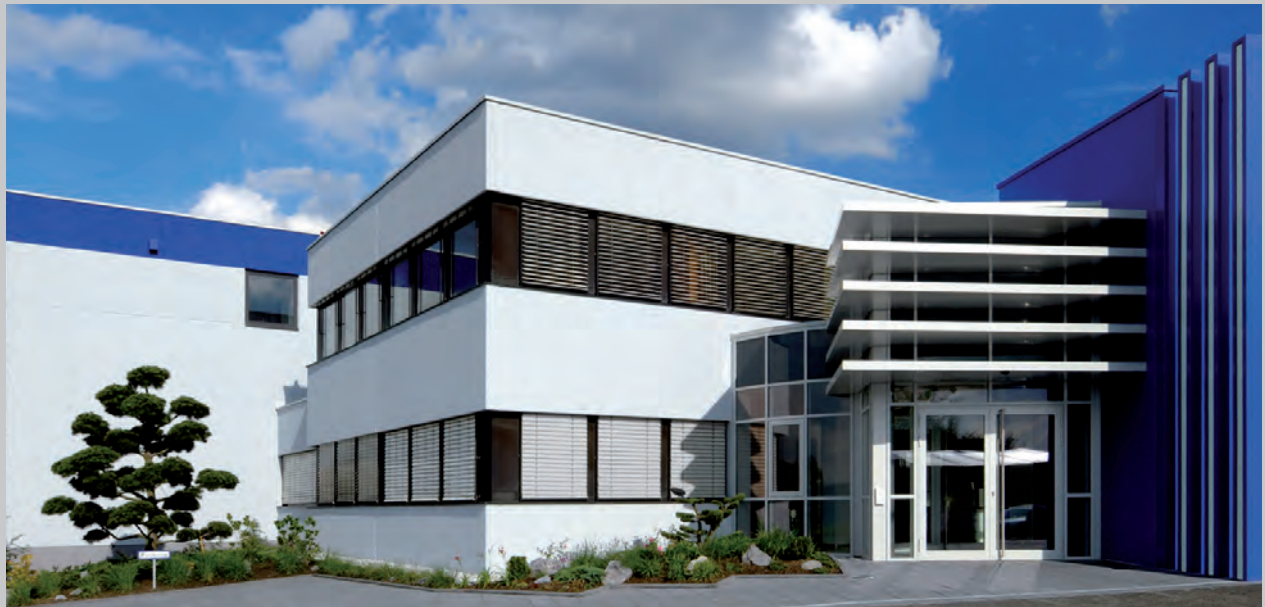
foyer of the company
