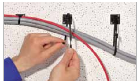
Q Ties can be used for temporary and final cable assembly.
