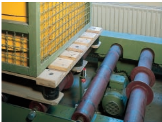
Proximity Sensor in a conveyer application.
