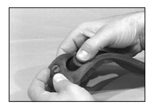
5.02 Install end seal on cable and put one wrap of vinyl tape around center of end seal.
