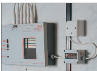
Ready boxed protector (here an ESP 240-5A/BX) installed on the fused connection (spur) to an alarm panel
