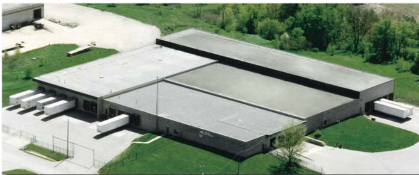
Hammond North American Distribution Centre
