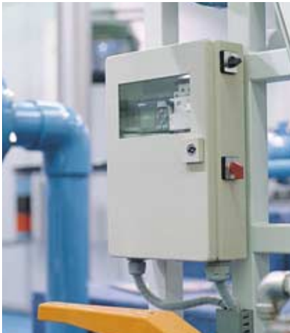
Other components where the LED or text display needs to be visible can also be accommodated behind the viewing windows.
