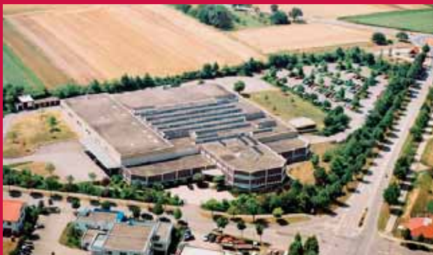
Cooper Hand Tools Besigheim, Germany
